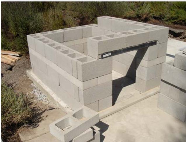
2.1 Angle iron supports the fourth block course.
