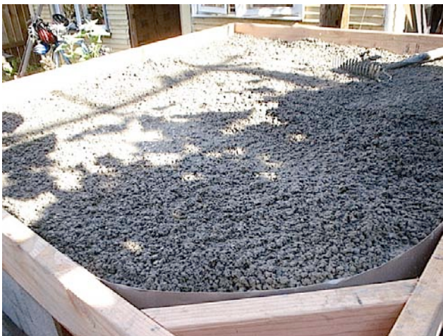
4.5. Insulating concrete on top ready to cure.
