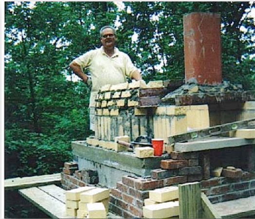
12.1. Refractory flue liner.
