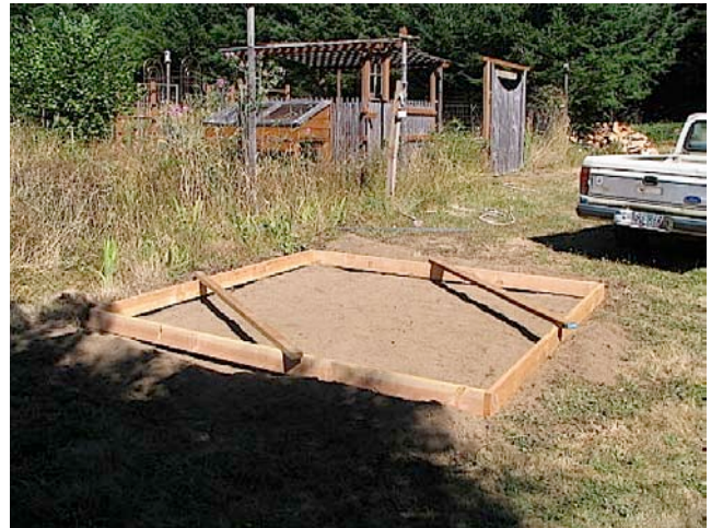
1.8. 2"x4"s hold the form square and plumb.
