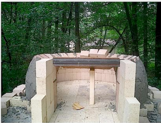
8.1. An angle iron framed opening. Note the lack of a reveal for the door jam (don't do this).
