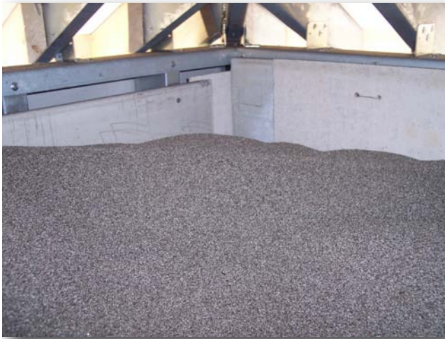
13.4 Loose vermiculite fills a walled enclosure.
