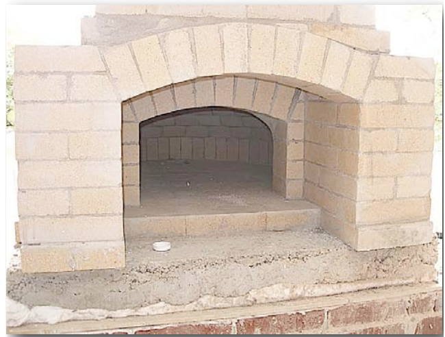
11.3. Different style brick arch with setback.
