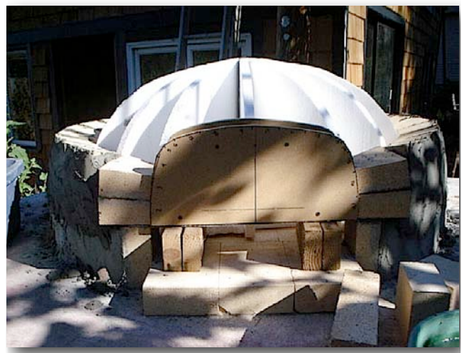
8.4. A form shapes oven opening.
