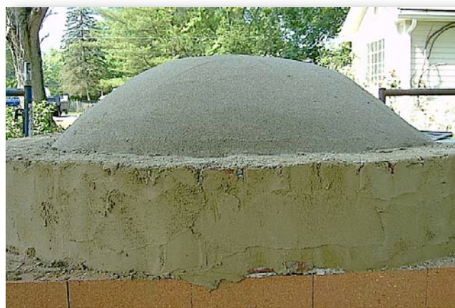
6.4 Sand form inside first course for bricks.
