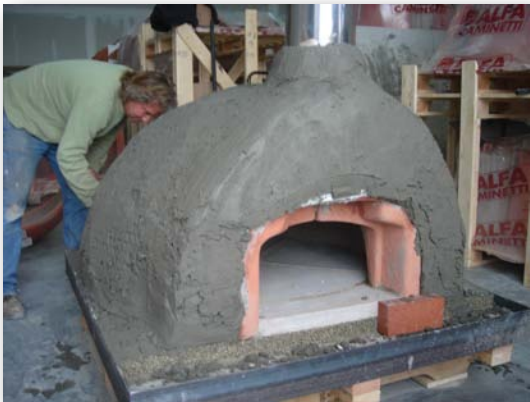
15.5 Rough coat of stucco on wire lathe.
