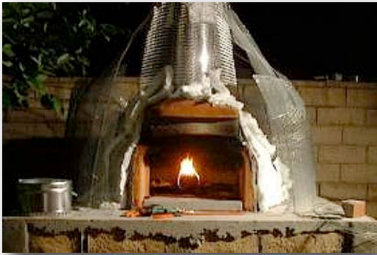
15.4 Rebar and lathe shape the Igloo.
