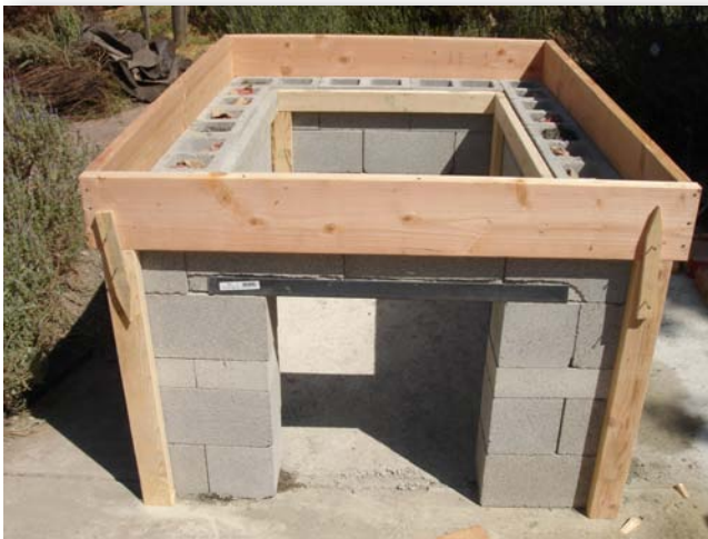
3.5 Form sides held in place with 2"x4"s.
