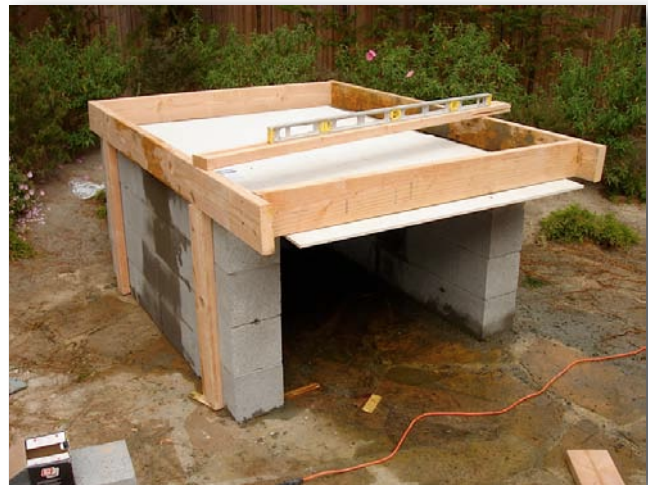
3.3. Hardibacker inside the side forms.
